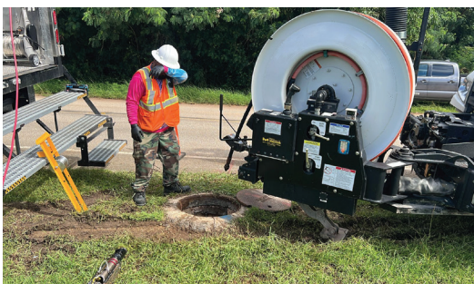
Wastewater Grout CCTV Inspection Truck
