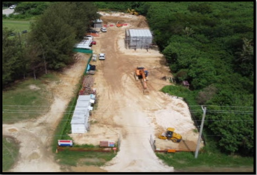
Dandan Water Tank Project Site
